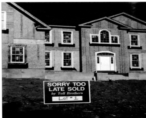
McMansion under construction, 2013 Westchester County, NY Fig 1. Examples of McMansion
